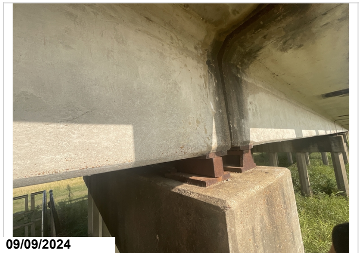
Bent 13, girder 4, back: has a shear crack measuring 6". 1LF CS3
