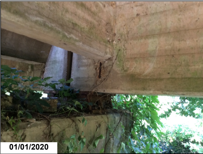
Spalls with rebar exposed to Girder 1 @ BOS 7.
