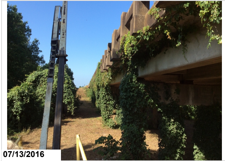
Heavy vegetation @ Bents 2 through 10 Right side of bridge.
