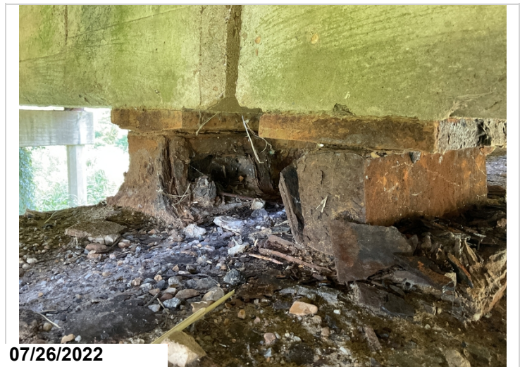
Bearings Rust, pack rust, and section loss to all moveable and fixed bearings.
