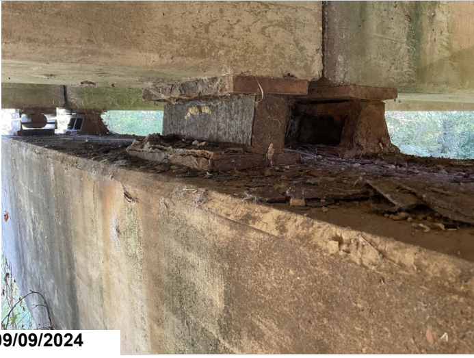
Bent 2, back: typical movable bearings have cs3 corrosion throughout with pack rust and section loss.
