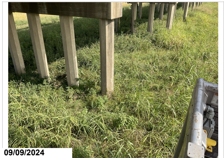
Bent 17, pile 5: has a spall. 1EA CS3
