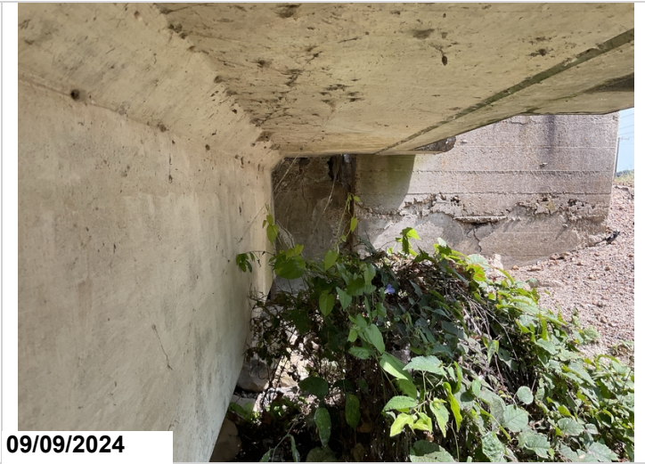
Abutment 2, right: has a large vertical crack. 1LF CS3
