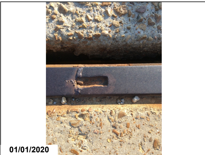
Span 14 - Crack in road iron at End of span.
