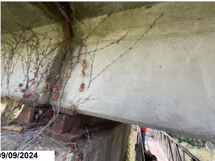
Bent 07, back, girder 1, left: has an 8" shear crack from the bearing area. Not mirrored on right. 1LF CS3
