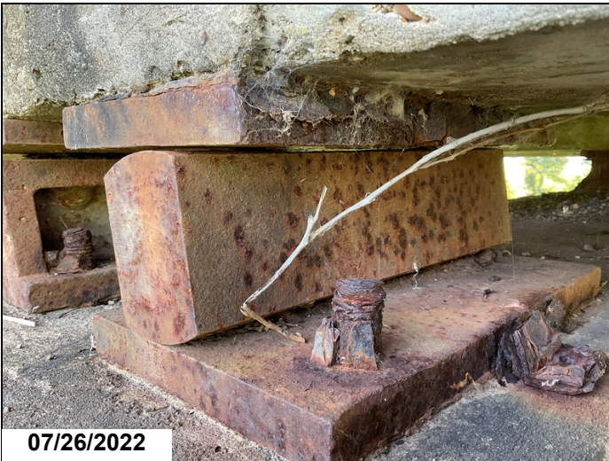
Moveable Bearings are NON-BEARING at: Bent 2 - Bearings 1 & 4. Bearing 1.
