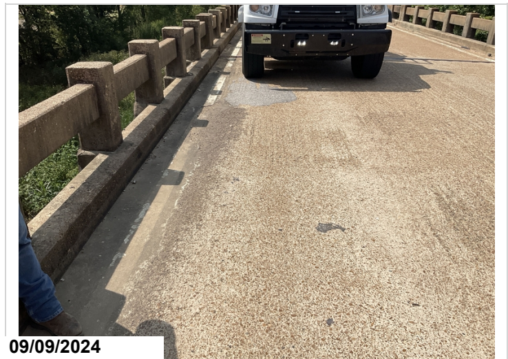
Span 36, right. Large spall
