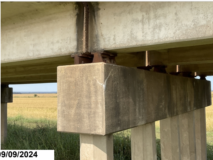
Bent 23, ahead, right, cap: has a diagonal efflorescent crack with buildup. 1LF CS3
