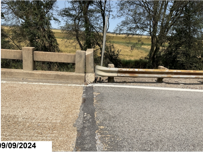
Abutment 2, left, end post at wing wall: has broken away. The right end is similar
