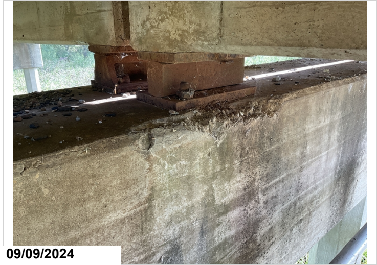
Bent 25, back, under bearing 3, cap: has a 2' spill. 2LF CS3
