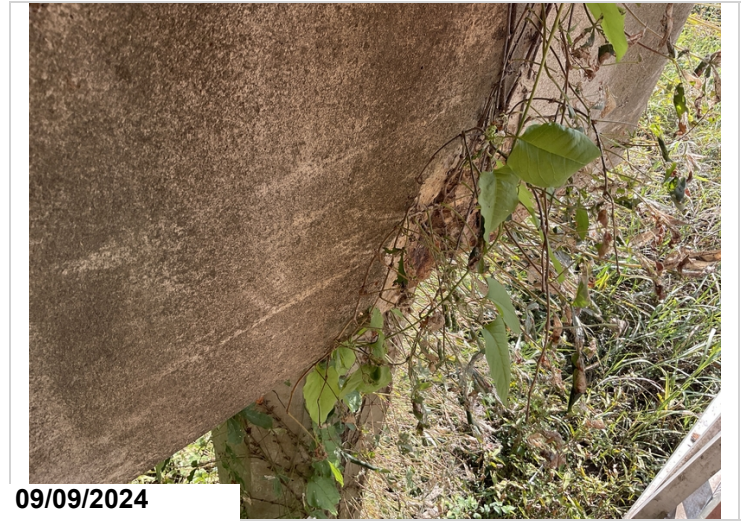
Bent 09, right, back, over pile 5: has a spall with exposed rebar. 1LF CS3
