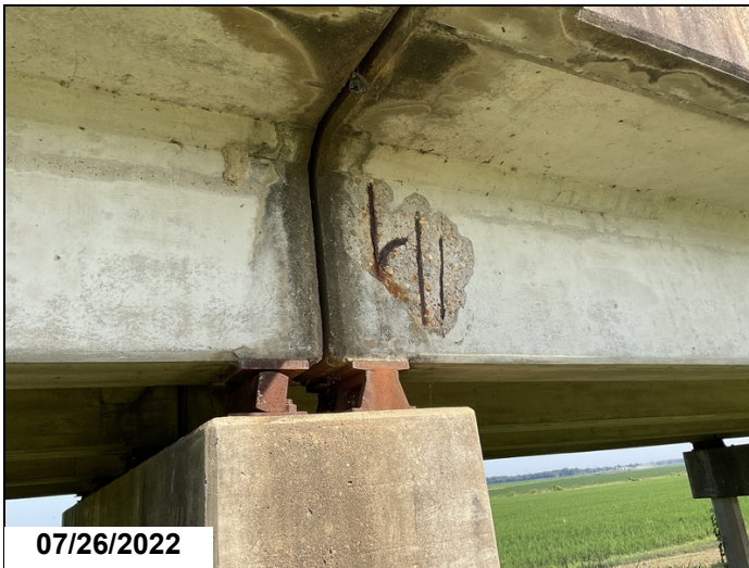
Concrete Girders Spalls with rebar exposed at Spans 3 thru 8, 11 thru 13, 15 thru 17, 20 thru 26, 28, 32. Girder 4, beginning of span 12.
