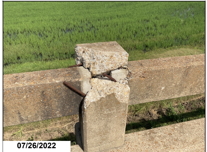
Collision damage to concrete bridge rail post @ Span 23 Left side.
