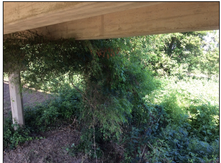
Tree growing under Left side of bridge @ Span 12.
