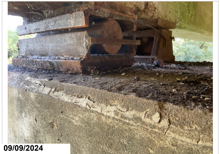
Bent 2, back, bearings 1 and 4: are non bearing. 2EA CS3
