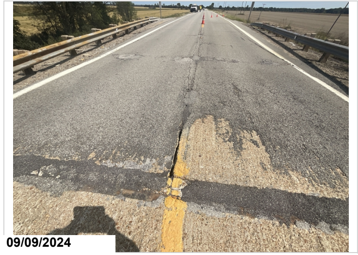
Abutment 2 approach voids
