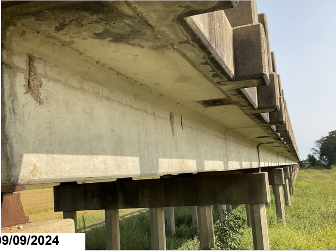
Span 13, girder 4, right: has small spalls with exposed rebar. 3LF CS3
