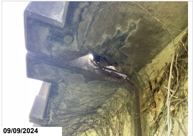
Bent 4, left, back, overhang: large spall at joint armor resulting in exposed rebar. 2sf cs3
