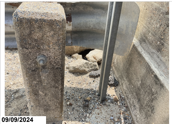
Abutment 2, both sides of the approach have voids
