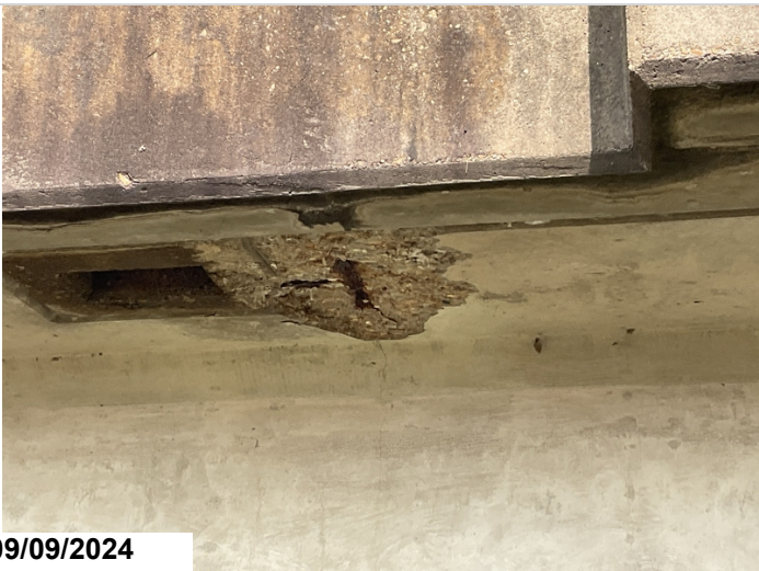
Span 12, right, 1lf cs3
