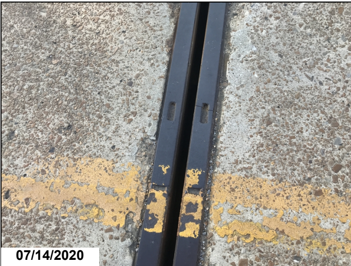
Span 3: Broke road iron @ End of span.
