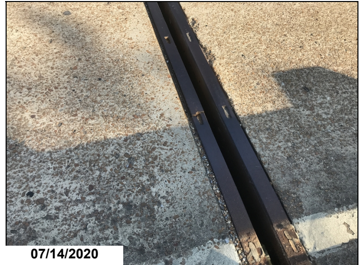
Span 27: Broke road iron at End of span.
