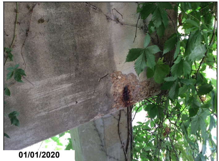
Spall with rebar exposed to cap @ Bent 9 backside above Pile 5.
