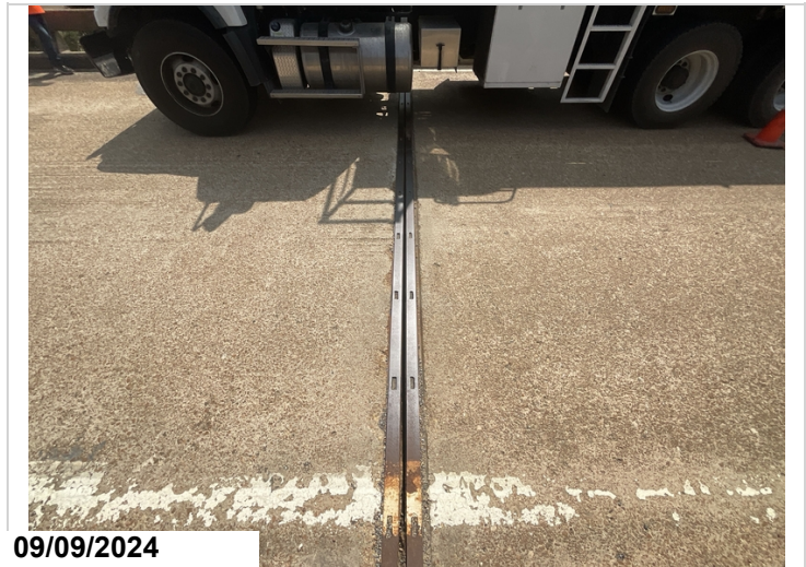
Bent 35: typical broken armor 15LF CS3
