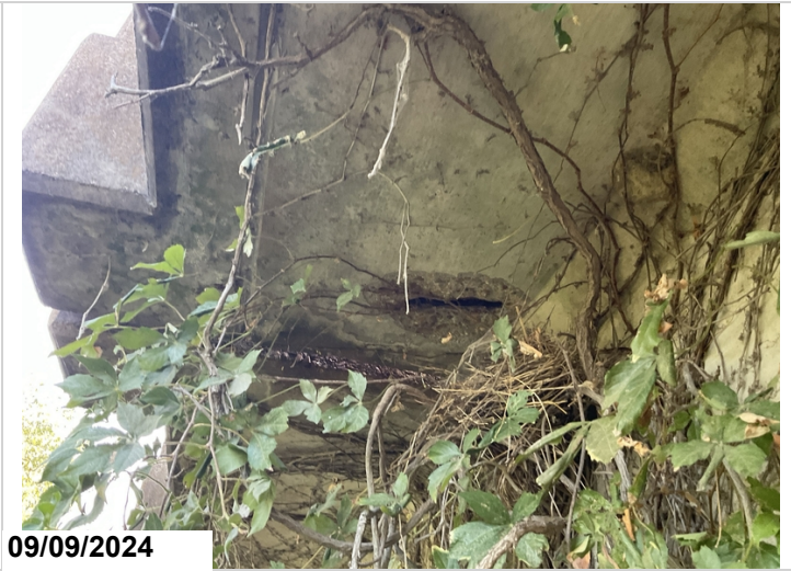
Bent 3, back, left, undersurface. Spall with exposed reinforcing steel. 1sf cs3 Span 5, right: 1sf cs3 Bent 6 left, back. 1sf cs3
