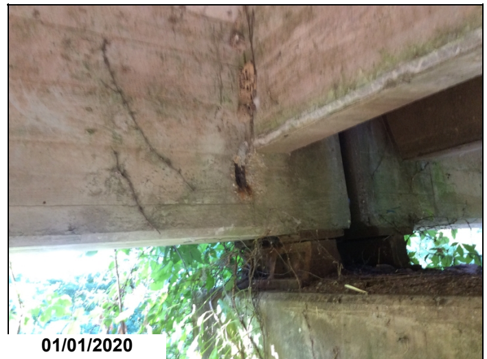
Spalls with rebar exposed to Girder 4 @ BOS 6.
