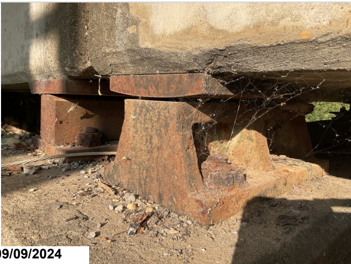
Bent 1, ahead, fixed bearings: pack rust has jacked the bearings up 1/8" all the way across.
