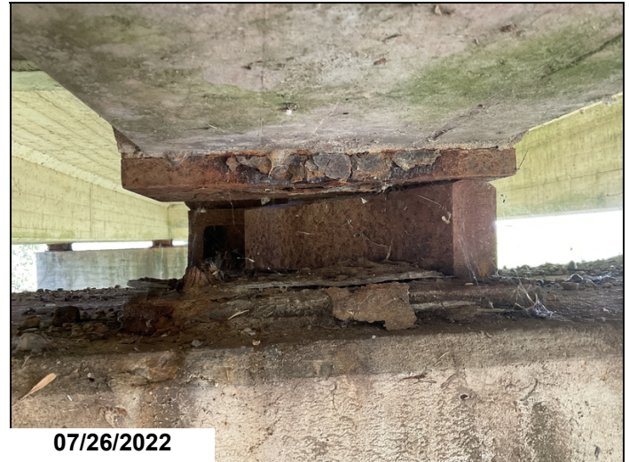
Moveable Bearing 3 at end of Span 8 has rotated out from under girder.
