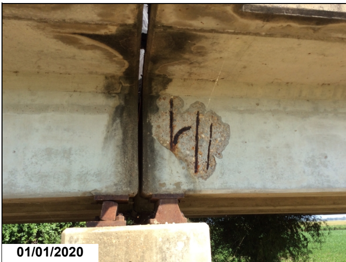
Large spall with rebar exposed to Girder 4 @ BOS 12.
