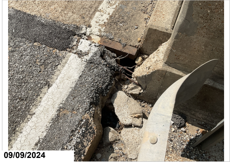
Abutment 2, left: Spalling on the headwall has caused a hole in the left shoulder. Right side is similar. 1LF CS3
