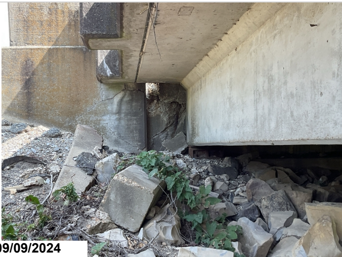
Abutment 1, left: has a large spall where the wingwall end post has broken. 2LF CS3 exposed rebar, 4LF CS3 crack
