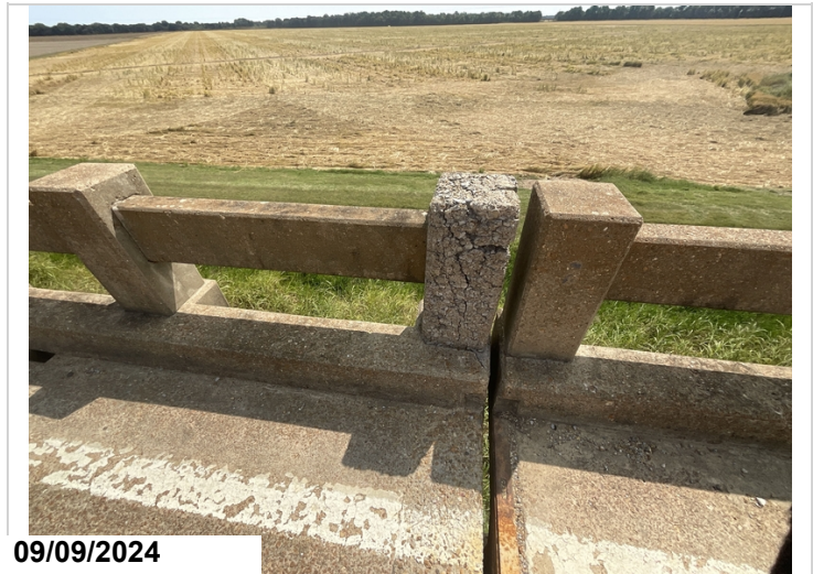
Bent 17, right, ahead: Heavy deterioration to the post. 1LF CS3
