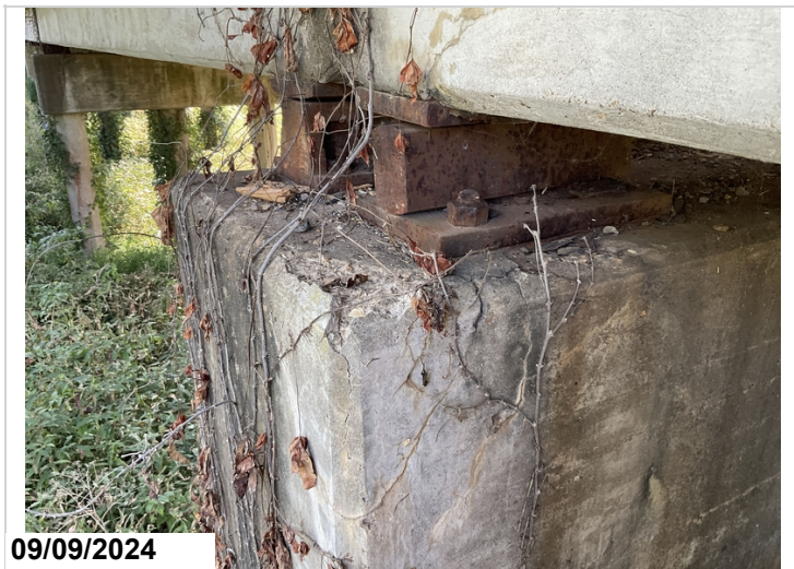
Bent 07, left, back: spall at cap end. 2lf cs3
