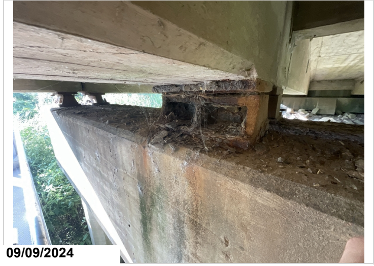
Typical fixed bearings have corrosion with section loss throughout
