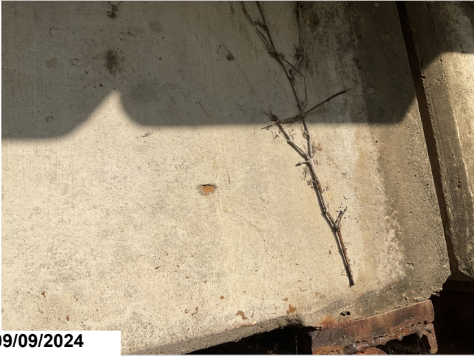
Bent 2, back, girder 4: typical hairline cracks at the girder ends
