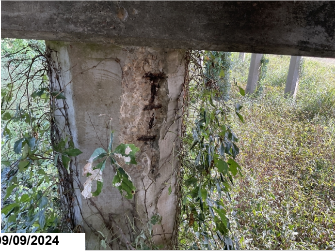
Bent 9, pile 2, back: has a spill with exposed rebar. 1EA CS3
