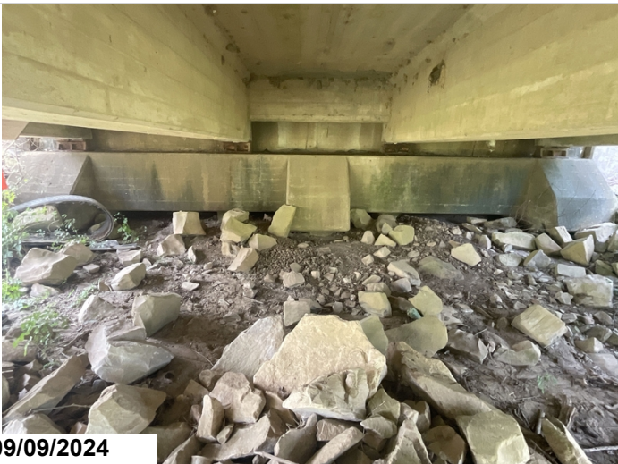
Abutment 1: has minor scour with 2 piles exposed. 16LF CS2
