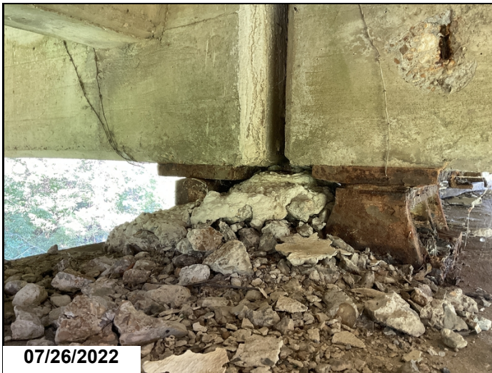
Span 6 - Concrete from Deck repair blowout restricting movement of Moveable Bearing 2 at Bent 6.
