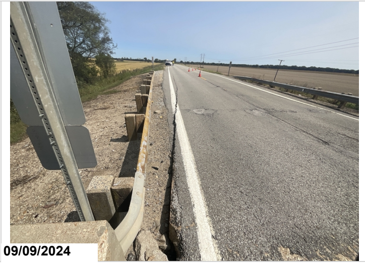
Abutment 2, approach voids
