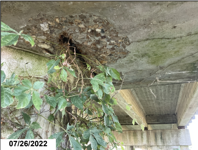
Concrete Caps Spalls with rebar exposed at Bents 4, 9, 23, 25 & 32. Bent 4 between piles 1 & 4.
