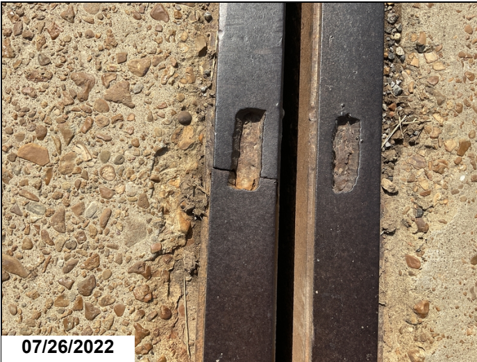
Cracks welds or broken/loose road iron at: Span 2 - Beginning of span.
