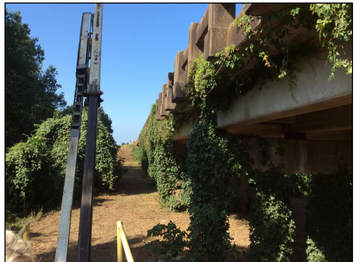
Heavy vegetation @ Bents 2 through 10 Right side of bridge.
