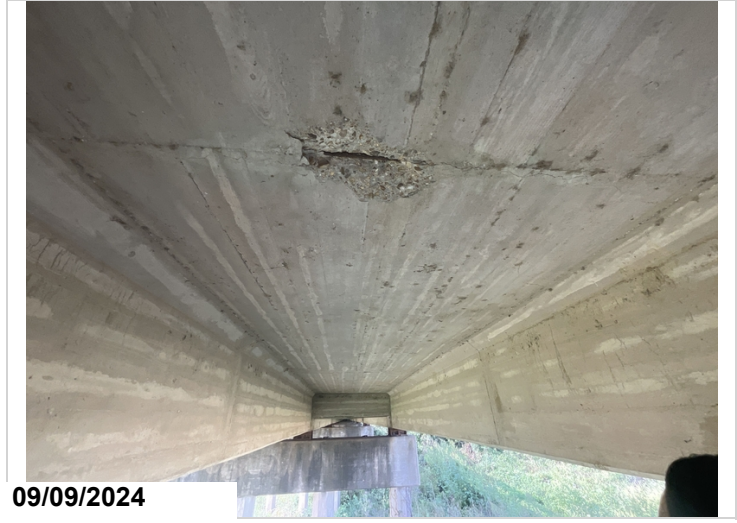
Span 13, bay 1: has exposed rebar. 1sf cs3 rebar
