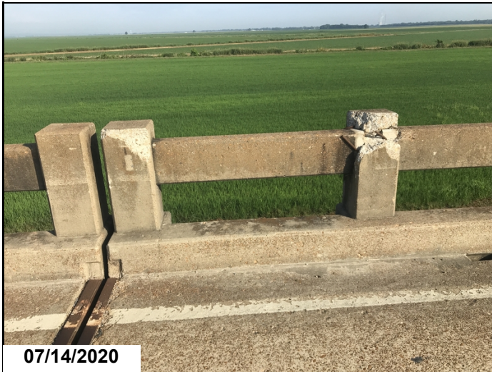
Collision damage to 1st & 2nd concrete post on Left side @ Span 23.
