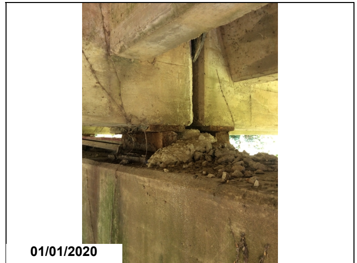
Span 6 - Concrete from deck repair blowout restricting movement of Bearing 2 Bent 6.
