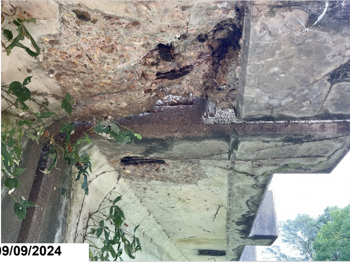
Bent 31, right, back has a large spall that is nearly 8" deep with heavily corroded rebar. 1sf cs3 spall, 1sf cs3 rebar. Ahead this location 1lf cs3 rebar
