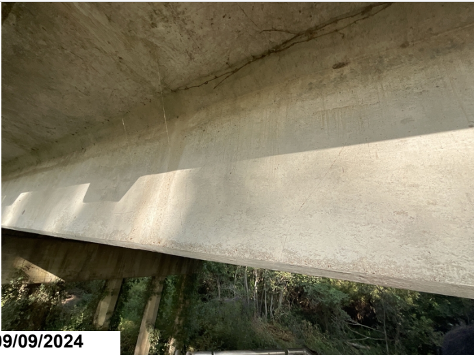
Typical girders have hairline flexure cracks at midspan.
