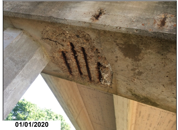
Spalls with rebar exposed to bottom of Cap @ Bent 23.
