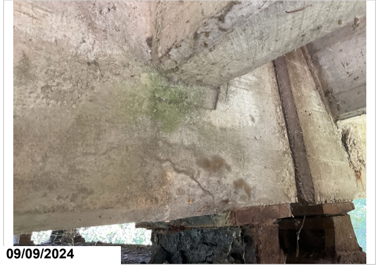
Bent 7, back, girder 2, right. 8" shear crack coming from bearing. This crack is mirrored on the left side
