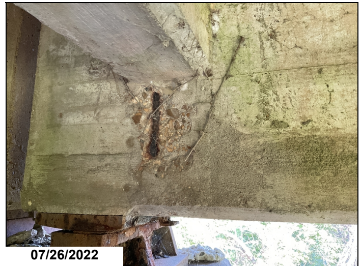
Concrete Girders Spalls with rebar exposed at Spans 3 thru 8, 11 thru 13, 15 thru 17, 20 thru 26, 28, 32. Girder 1, Beginning of span 7.
