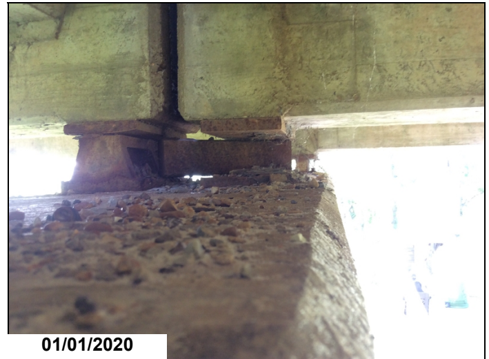
Bent 8 - Moveable bearing 3 (back side) at End of span has rotated Ahead out of place.
