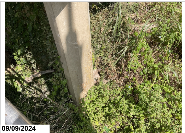
Bent 35, pile 5: has a spall. 1EA CS3
