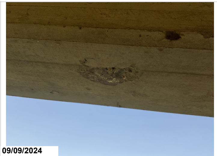
Bent 24, back girder 1: has a spall. 1LF CS3
