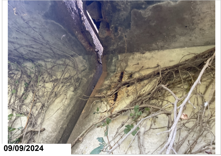
Bent 04, back, girder 1: has a spall with exposed rebar. 1LF CS3
