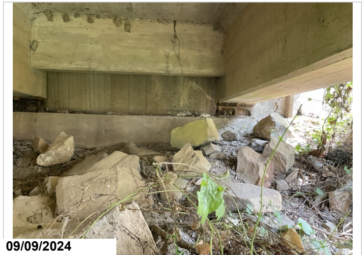
Abutment 2: typical diagonal efflorescent cracks. 8LF CS2
