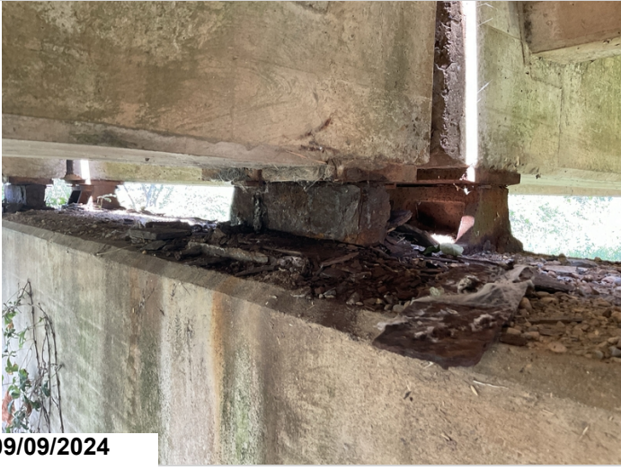
Bent 29, back, bearing 2: is non bearing. 1EA CS3
