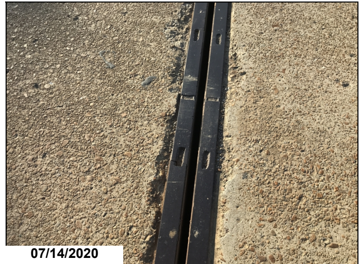
Span 2: Broke road iron @ Beginning of span.
