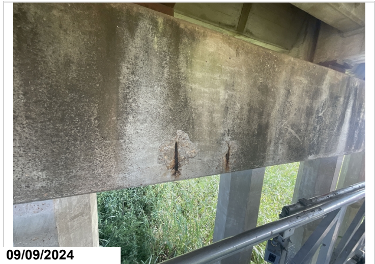
Bent 23, back, cap: has a spill with exposed rebar. 2LF CS3
