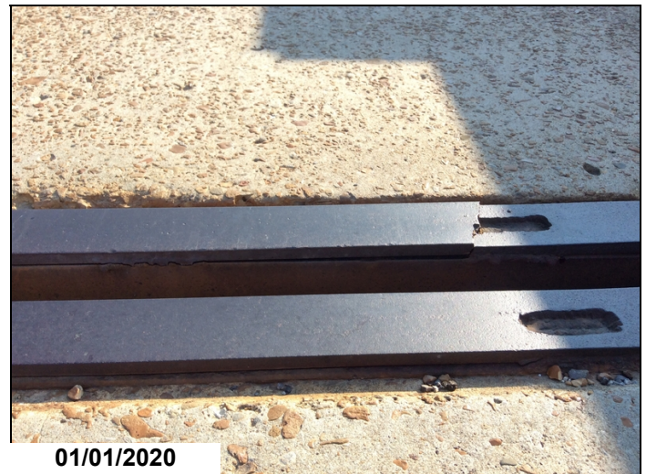
Span 33 - Broke road iron at Beginning of span.
