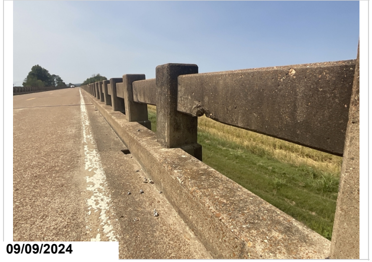
Span 26, left: typical spalling and cracking to guard rail.
