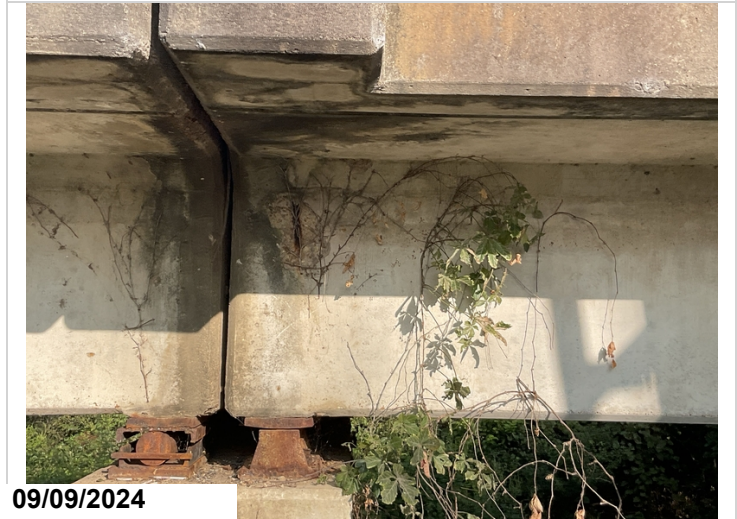
Bent 2, ahead, girder 4: spall with rebar. 1LF CS3
