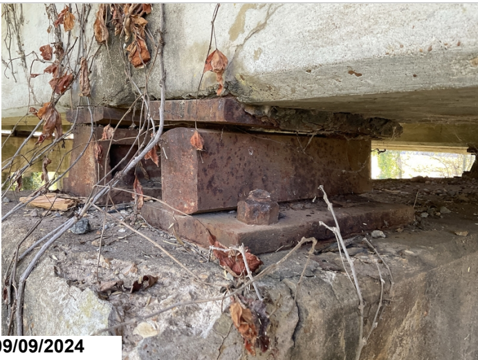
Bent 7, back, bearing 1: is non bearing. 1EA CS3
