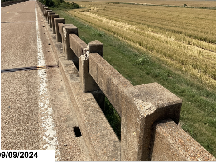
Span 23, left: spalling throughout.
