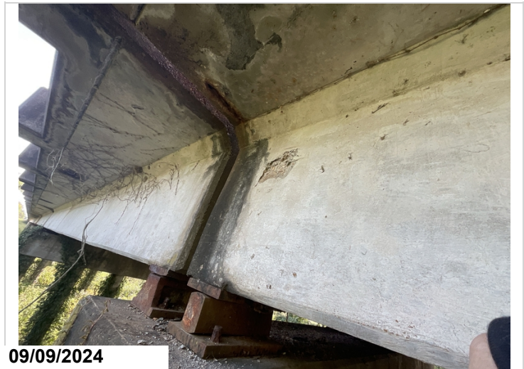
Bent 05, girder 1, left: has a minor spall. 1LF CS3
