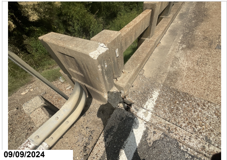
Abutment 1, left: the wing wall has broken away similar to abutment 2.
