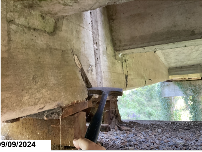
Bent 5, girder 1, right: has a void in the end 1.5" deep and 6" tall above the bearing
