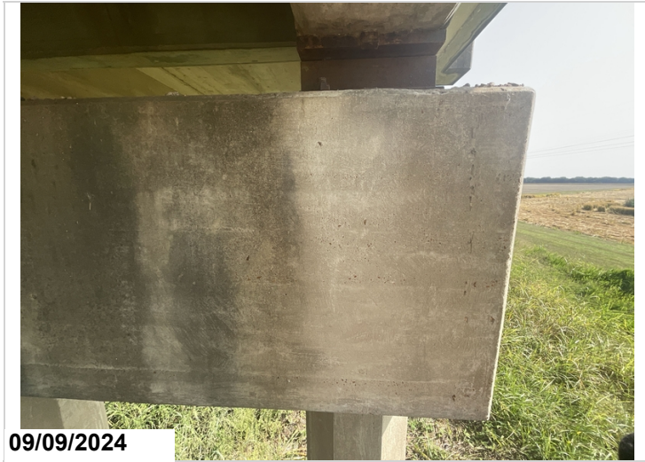
Typical cap crack
