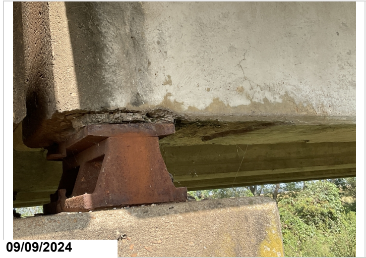
Bent 28, ahead, girder 4. Deterioration to girder end for 3ft. 3lf cs3
